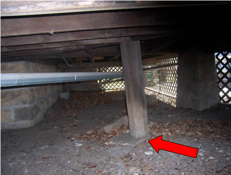
Front porch posts are poorly supported – they do not rest on a proper footing
