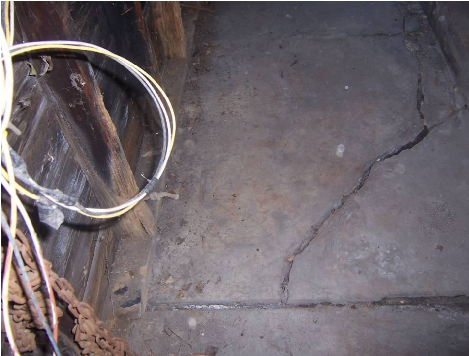
Garage slab and foundation have settled, and walls are not properly supported
